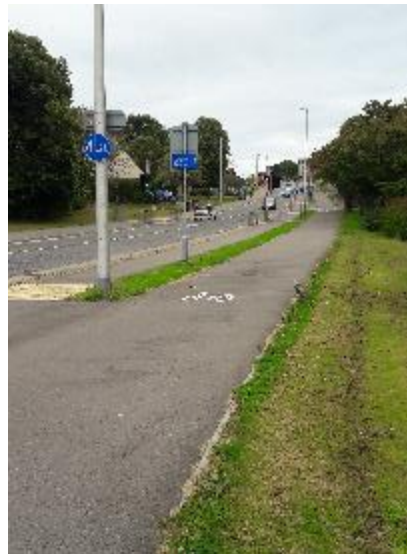
Photo 5 - Segregated section on Tillydrone Road
